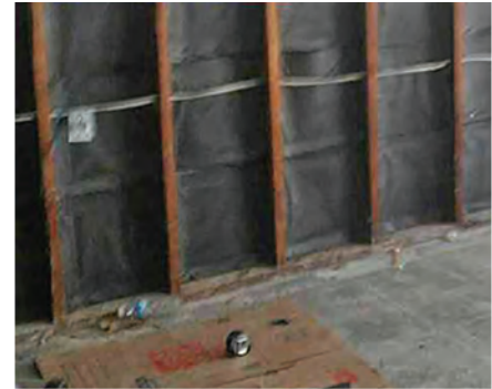
FIGURE 5 (ABOVE LEFT) AND PHOTO 7 (RIGHT) Drainage Mat. A drainage mat with a filter fabric is installed directly against the interior of the brick veneer with the filter fabric facing inward. This approach eliminates the need for the “wedges,” but it requires the use of a thicker layer of SPF. Photo courtesy of Joseph Pauwels. FIGURE 6 More Spray Polyurethane Foam. The SPF needs to “catch” the stud cavity, filling it at least 3 in. (75 mm) thick to provide the racking resistance. Once again, we have to coat all the interior surfaces with acrylic latex paint prior to the installation of the interior gypsum board.
