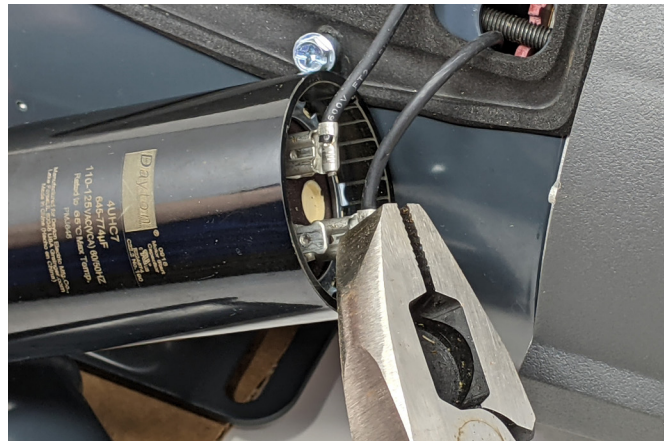
Figure 5. Electrically insulated pliers are used to remove the wiring connectors from the capacitor tabs. Do not use your fingers as the capacitor might be holding a charge.
