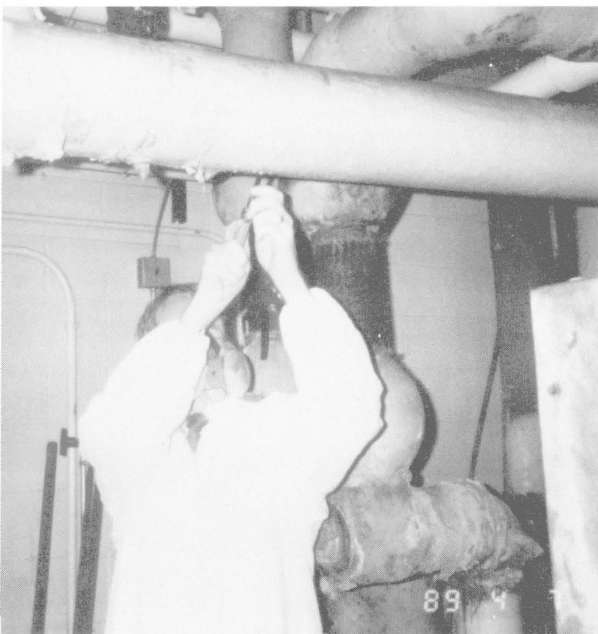
A properly trained and protected building inspector collecting a bulk sample of suspected asbestos-containing thermal system insulation.
