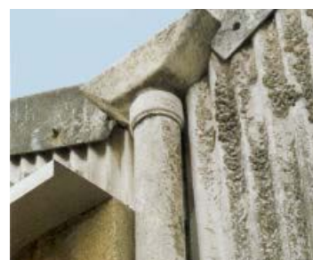
Figure 35 Asbestos cement downpipe
