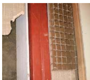
Figure 21 AIB column fire protection in CLASP building
