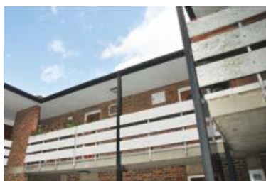
Figure 18 AIB exterior panel on open walkway
