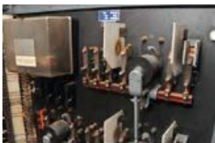
Figure 50 Open electrical switchboard with asbestos flash guards
