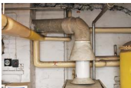
Figure 34 Asbestos cement boiler flue
