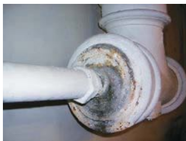
Figure 30 Amosite and chrysotile packing on waste pipes
