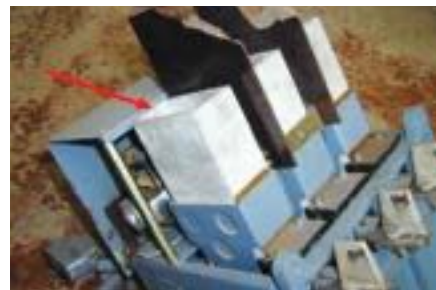
Figure 49 Electrical switchgear with asbestos flash protection
