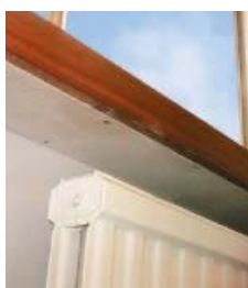
Figure 20 AIB panel between radiator and window
