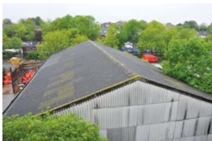
Figure 32 Asbestos cement roof and cladding
