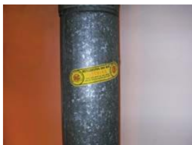
Figure 43 Metal clad gas flue containing chrysotile lining
