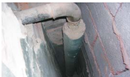
Figure 9 Lagged pipe in wall cavity
