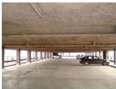
Figure 7 Sprayed limpet on car park roof
