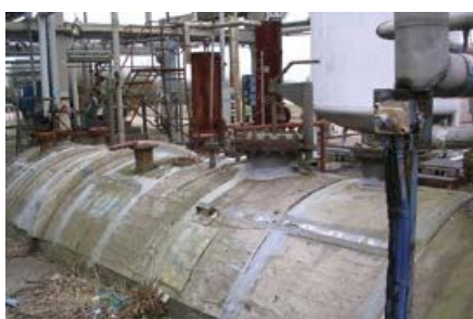
Figure 12 Lagging on large petrochemical vessel
