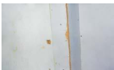
Figure 24 Chrysotile paper on fibreboard boxing
