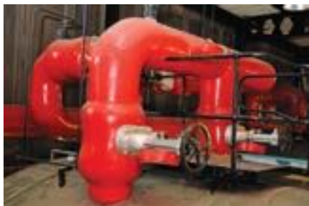
Figure 48 Asbestos-insulated supply pipes
