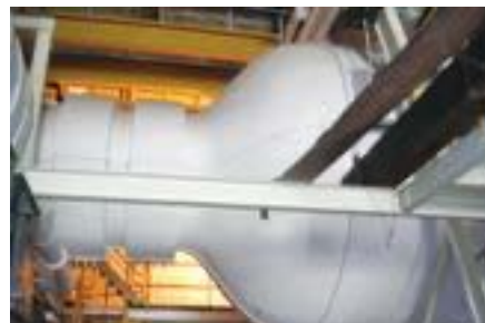
Figure 51 Vessel clad in amosite insulation
