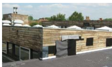
Figure 23 AIB fascia panels with wood effect finish
