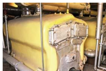
Figure 13 Amosite lagged boiler with hard plastic coating
