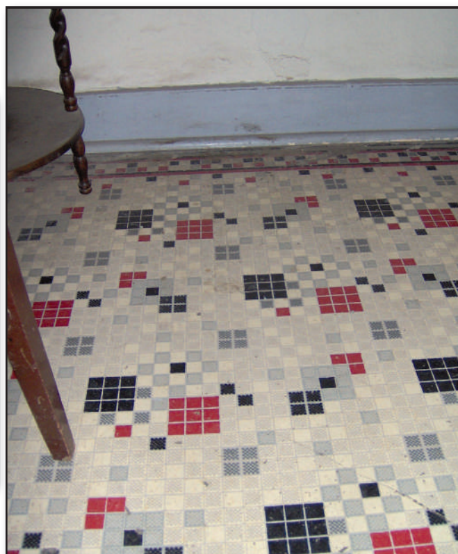
Figure 3—This linoleum flooring is holding up fairly well, but the printed pattern is scratched and worn.
