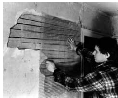
In this New Hampshire residence dating from the 1790s, the original plaster was a single coat of lime, sand, and horsehair applied over split lath. A one-coat repair, in this case, is appropriate. Photo: John Leeke.
