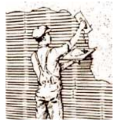
Plasterers applying rough and finish coats of plaster. Drawing: From the "Book of Trades."
