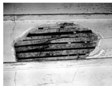
This beaded ceiling in one of the bedrooms of the 1847 Lockwood House, Harpers Ferry, West Virginia, is missing portions of plaster due to broken keys. Photo: NPS files.
