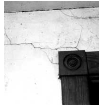
Stress cracks in plaster over a kitchen door frame can be repaired using fiberglass mesh tape and joint compound. Photo: NPS files.
