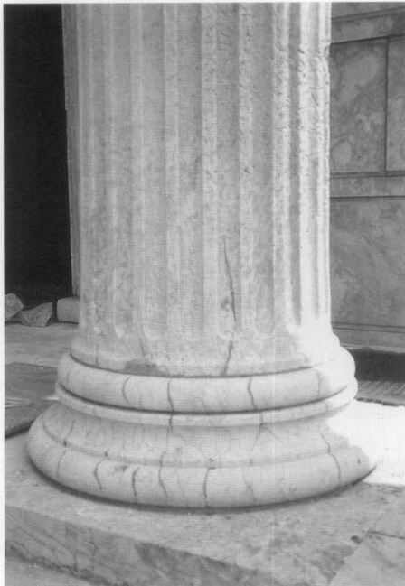
Fig. 10. The column base and plinths had extensive exterior cracks. The internal column cracks were detected by ultrasonic pulse velocity and impulse radar investigation techniques. Photo: Edmund P. Meade, P.E.
