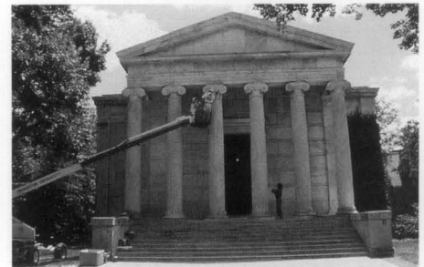
Fig. 13. The non-destructive evaluation of Whig Hall allowed the diagnosis of the condition of the masonry and the specification of a relatively low impact repair. Photo: Edmund P. Meade, P.E.
