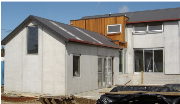
Panels installed on top of underground masonry retaining walls
