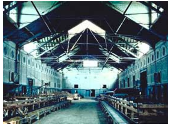
The interior of the barn in Shelburne, Vermont, is a magnificent space that included an overhead hay loft with tracks that allowed workers to drop hay to the floor below. Photo: NPS files.
