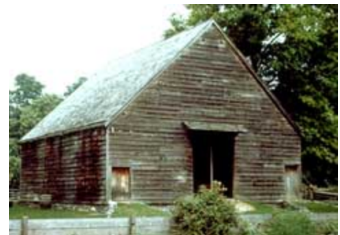
A gable roof, center wagon doors with pent roof, stock door at the corners, and horizontal clapboarding are all typical features of the Dutch barn.
